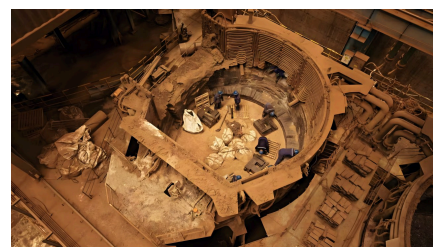
Electric furnace, 150 t: refractory materials, overall contracting.
